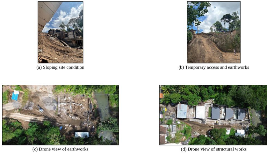
Figure 1. Case project documentation of the investigated structural works.
